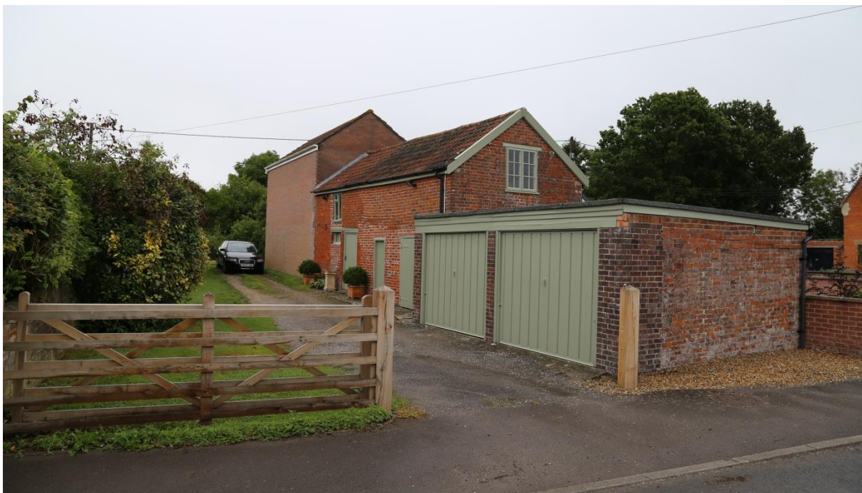
Restored property and outbuilding, Foster's Hill:
